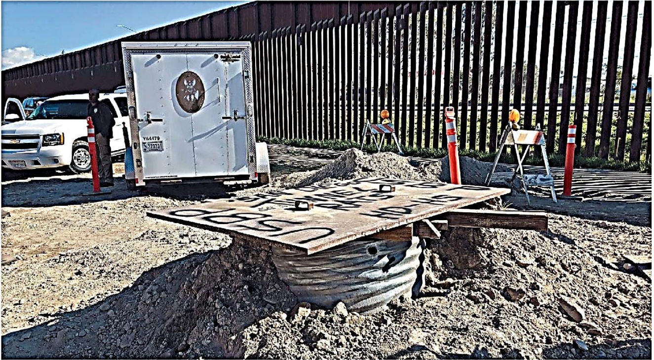
The tunnel is some 22 metres below the ground and equal to over 14 football fields long.
