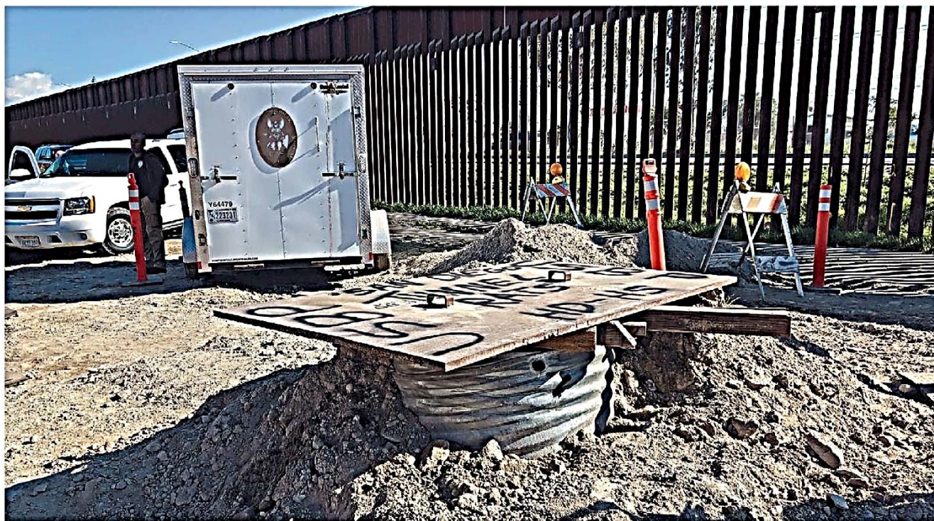
The tunnel is some 22 metres below the ground and equal to over 14 football fields long.
